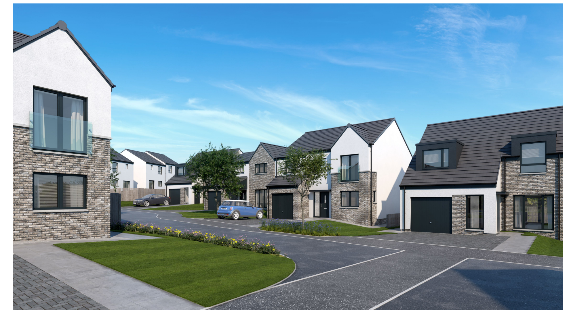
Street scene at Avant Homes development in Glenboig
